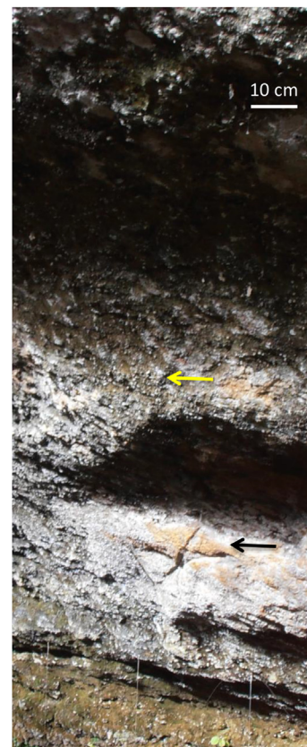
Fig. 1. Picture showing the walls of the Laugerie-Haute East shelter, Eyzies de Tayac-Sireuil, Dordogne, France. Efflorescences of white salts distributed heterogeneously are visible on the wall (upper part of the image, yellow arrow). Engravings are present below this area efflorescence (black arrow). (For interpretation of the references to colour in this figure legend, the reader is referred to the web version of this article.)
