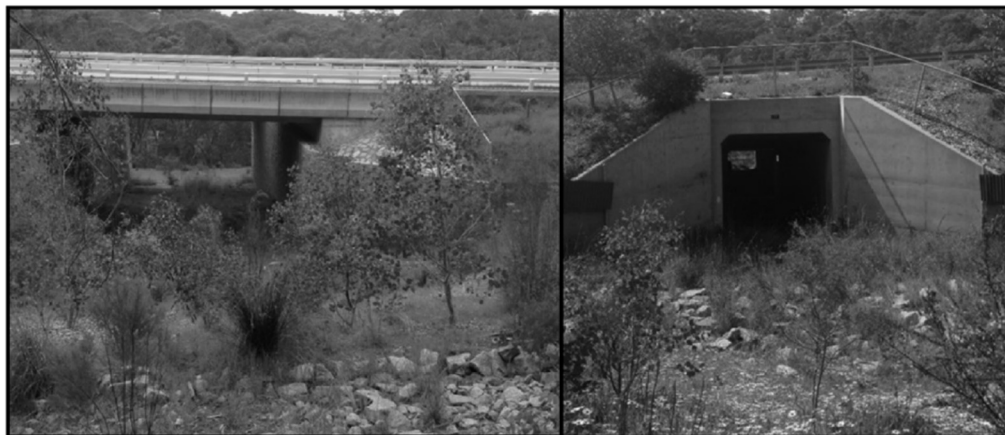
Fig. 1. Examples of one of the open-span bridges (left) and one of the box culverts (right) where bat movement was studied along the Calder Highway, in Victoria, Australia. Photos not to scale.
