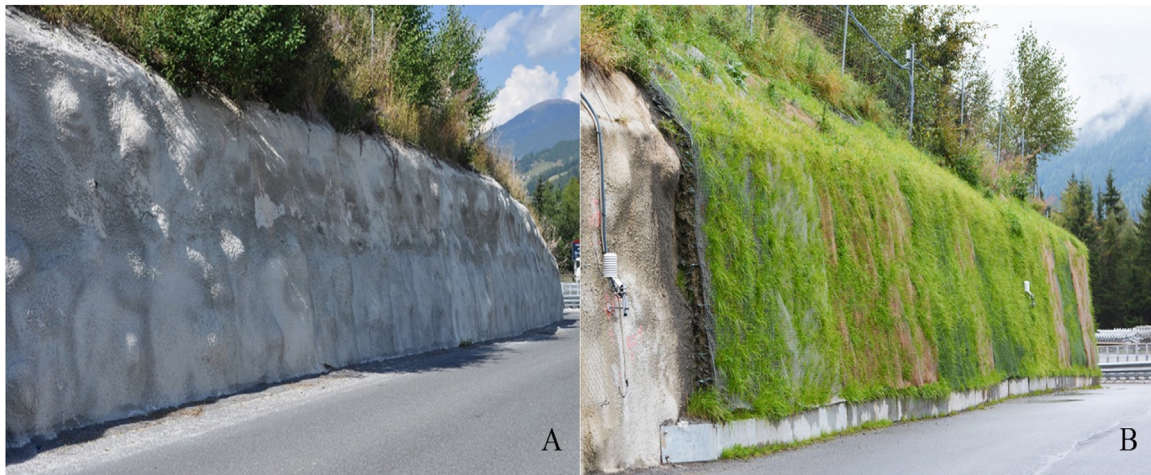
Fig. 1. Field experiment on the shotcrete wall along a highway exit. (A) Shotcrete wall without greenery system in May 2015 and (B) three months after installation in September 2015.
