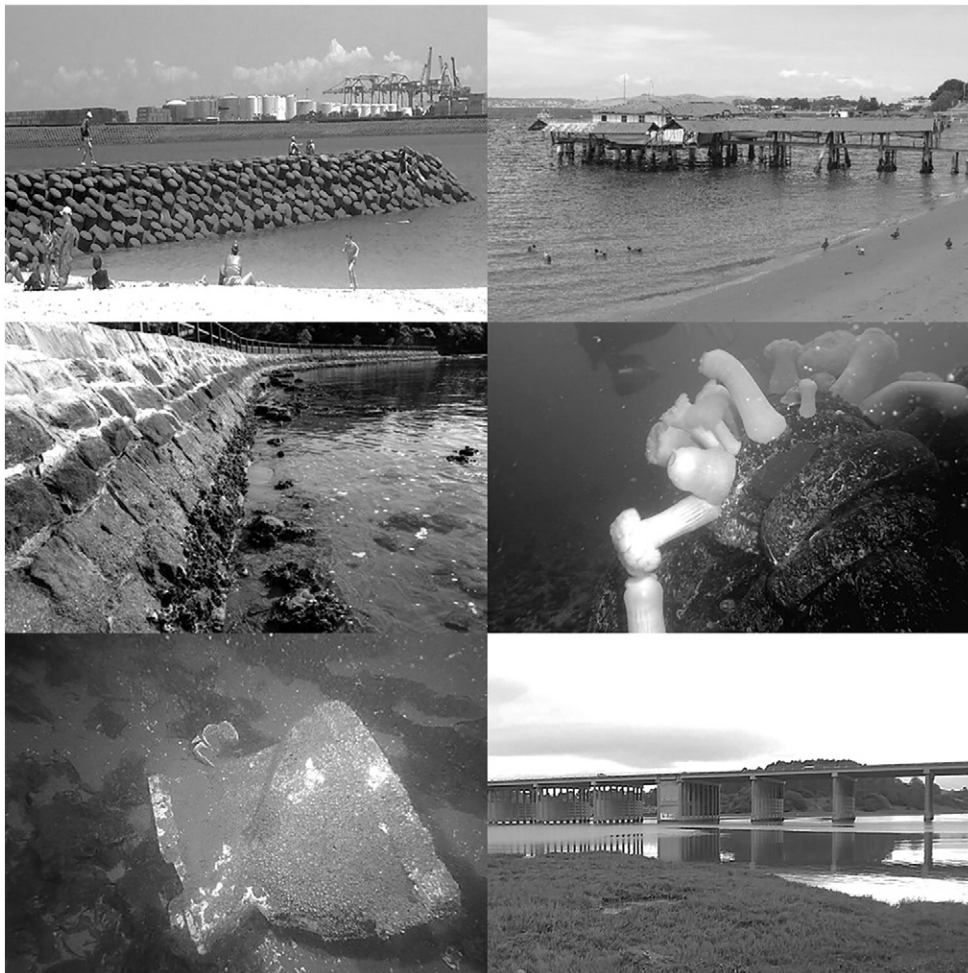
Fig. 1. Examples of artificial structures in sedimentary environments. From left to right: groyne a , pier a , revetment a , dumped appliance (toilet) b , tire reef b , and overwater causeway b . Photo credit: a E. Strain, b E.C. Heery.
