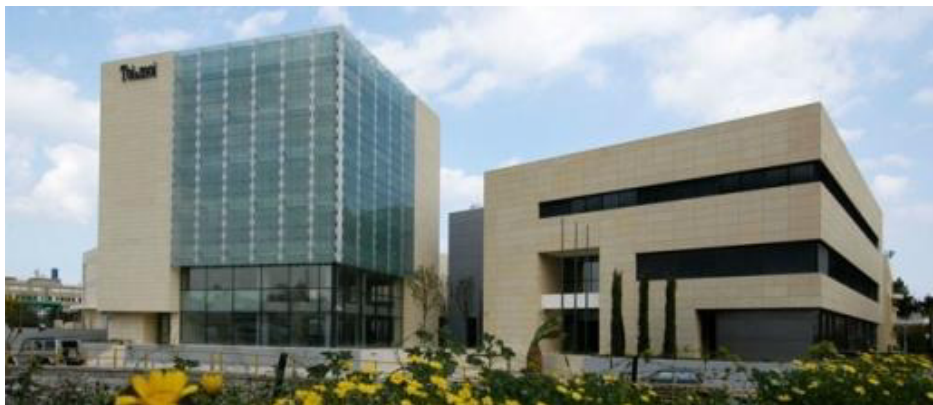
Fig. 1. The corner double skin façade that has been investigated.
