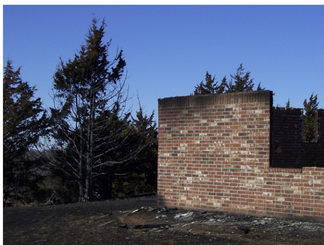
Figure 2. Wildfire damage in north-central Oklahoma in 2012. Note the proximity of eastern red cedars to the destroyed property. Photo credit: J.R. Weir.
