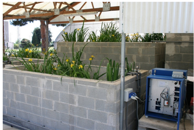
Fig. 1. Constructed wetland (CW) module and on-line analyzers connected to the inflow and outflow pipes of the CW.
