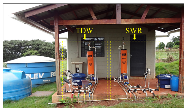
Fig. 1. Control head for two sets of pressurized systems, one for each water source. TDW: treated domestic wastewater, SWR: surface water reservoir.
