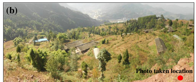
Fig. 4. Gaituping landslide. (a) An overview; (b) buildings at risk located at the right-front of the landslide; photo was taken above the landslide.
