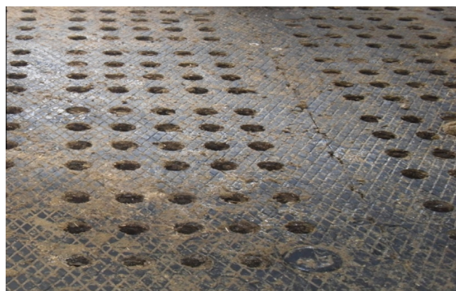
Fig. 3. Perforated concrete floor coated with a rubber mattress used in the experimental pens.
