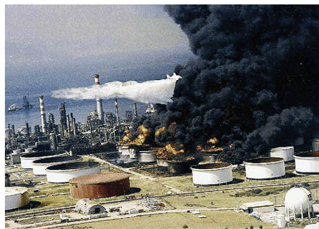
Fig. 2. Aerial view of Tupras refinery after the Kocaeli earthquake (Turkish Press, 1999).
