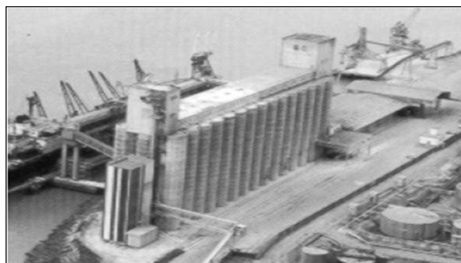
Fig. 2 – View of the Semabla cells and warehouse-A storage units before the explosion (Masson, 1998).
