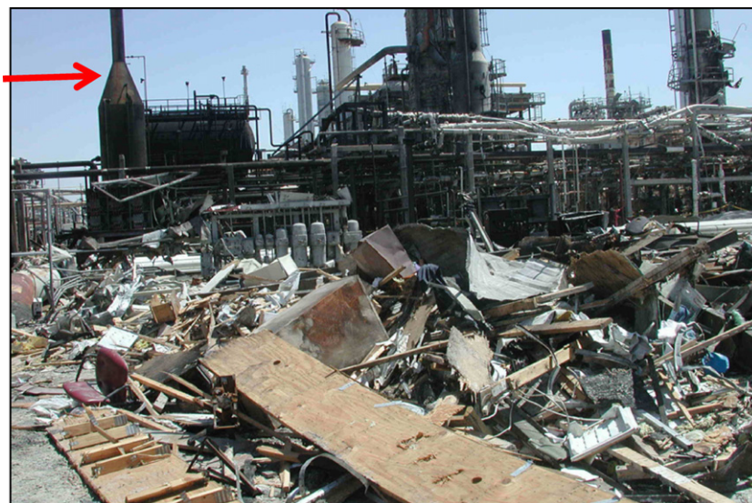
Fig. 1 – BP Texas City; destroyed trailers west of the blowdown drum (red arrow in upper left of the figure). (For interpretation of the references to color in this figure legend, the reader is referred to the web version of the article.) Original image from CSB (2007), Fig. 13.
