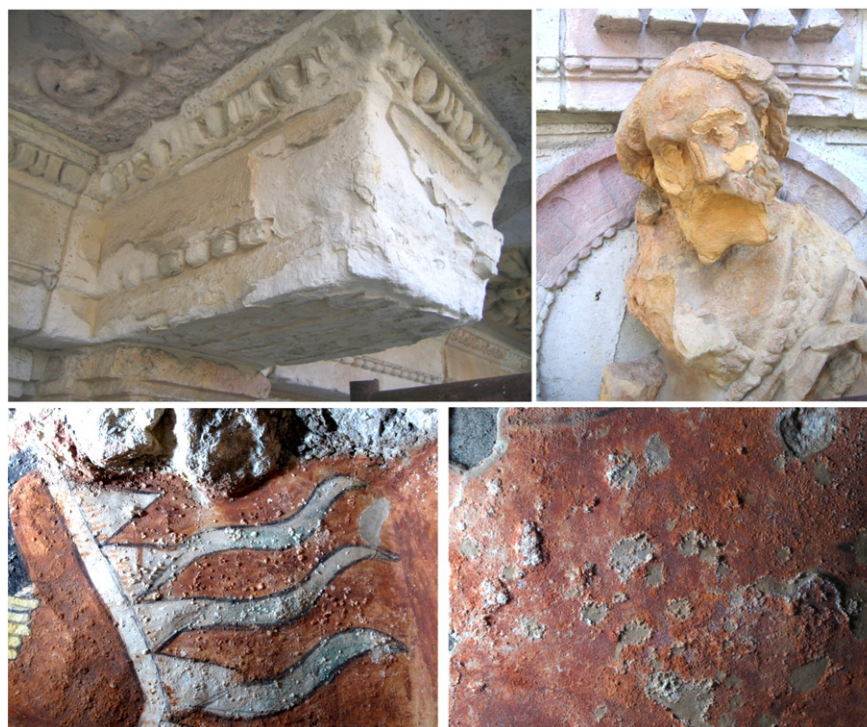
Fig. 1. Effects of salts crystallization on the surface of works of art. (Top row) 17th century limestone works (Angera stone) from the Ca' Granda Palace in Milan (Italy) showing delamination induced by salts in outdoor environment. (Bottom row) Mesoamerican wall paintings recently discovered in tombs located near Puebla (Mexico), where salts efflorescence causes flaking of the surface.
