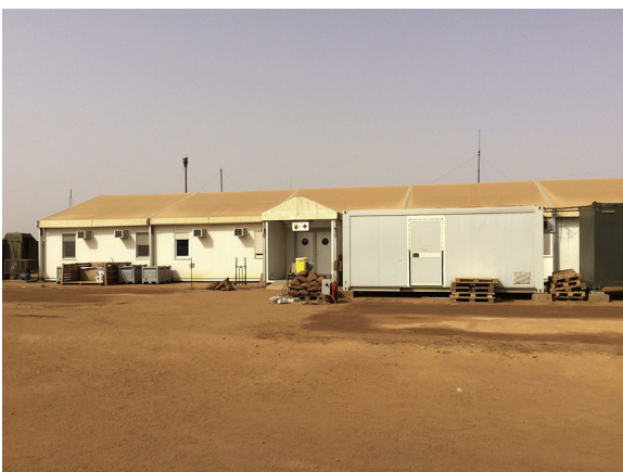
Fig. 1. Metallic and textile structure of the French Role 2+ in Gao, Northern Mali, during Operation Serval.
