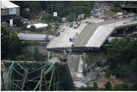
Fig. 1. Northern portion of the 35W bridge collapse. The majority of critically injured victims were extricated from the riverbank and area below the overhanging section of the bridge where the blue van came to rest. Overall debris field was >1 mile in length. Photo courtesy of the Minneapolis StarTribune – used with permission. (For interpretation of the references to colour in this figure legend, the reader is referred to the web version of this article.)
