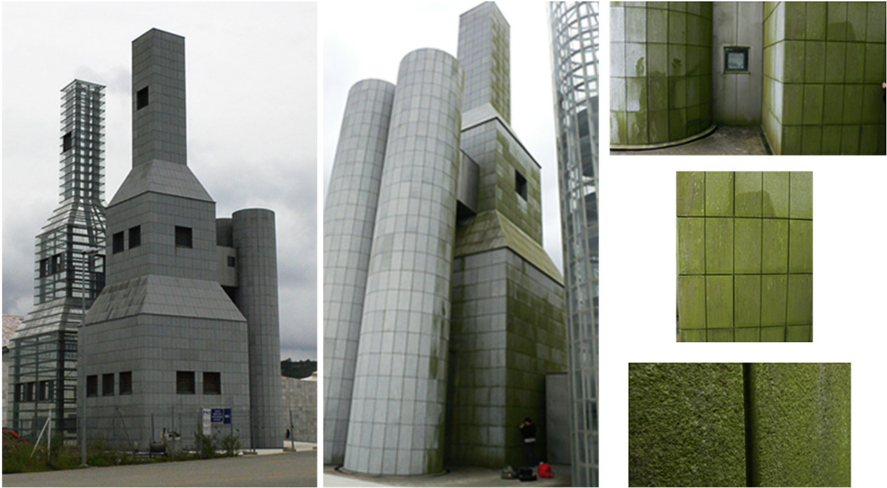
Fig. 1. The Hejduk Towers in the Cidade da Cultura de Galicia (Santiago de Compostela, Northern Spain) constructed with a ventilated facade and showing extensive phototrophic colonization (“greening”). The towers were built between September 2002 and February 2003. The granite used for the ventilated facades is Azul Extremadura with a sawn finish.
