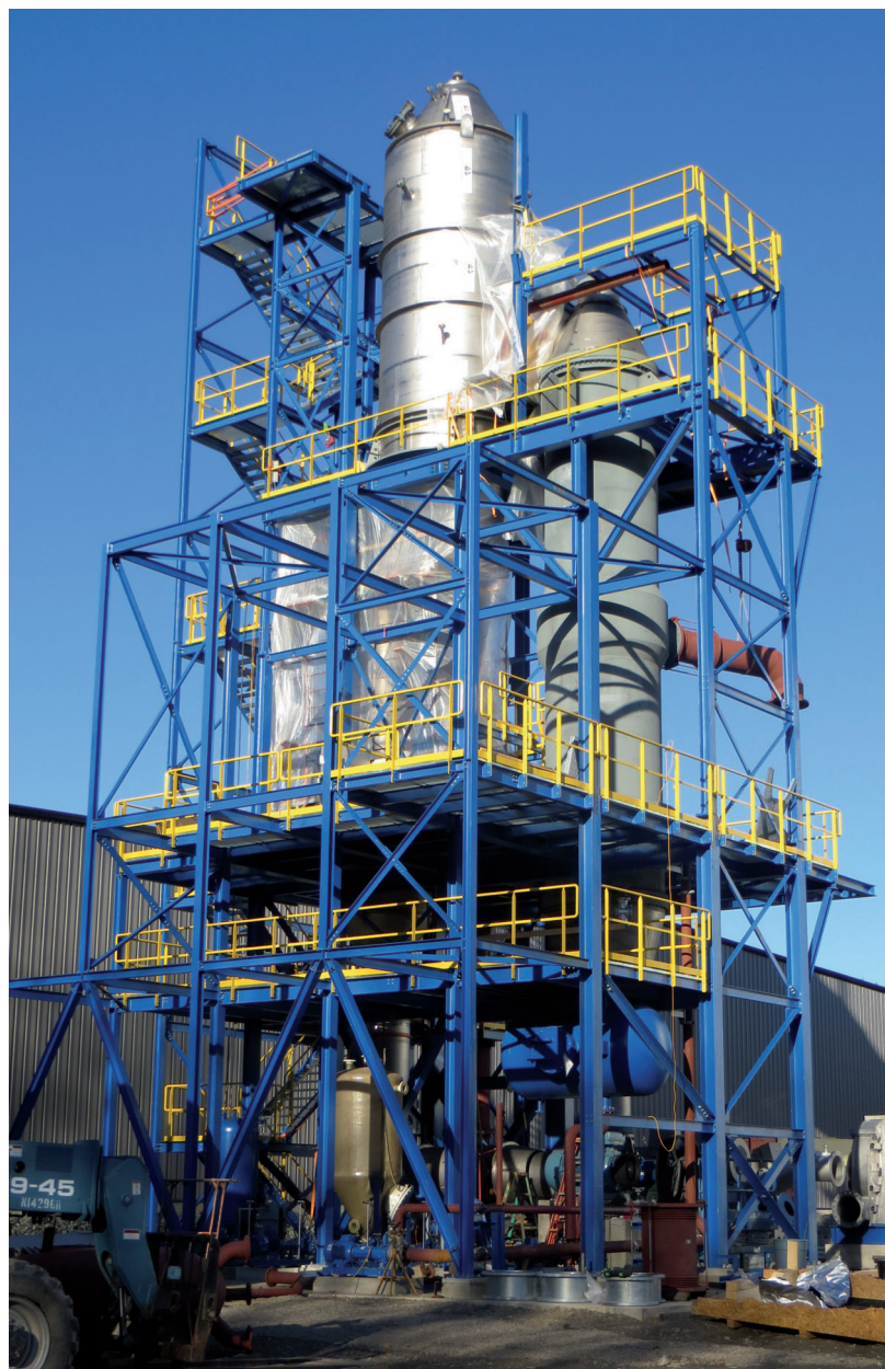
Figure 2. Evaporation tower in zero liquid discharge system. Image courtesy of H+E GmbH.
