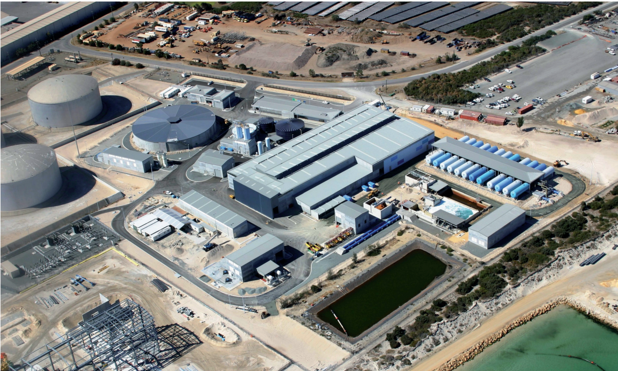
RO desalination installation at Perth, Australia (Courtesy of IDA).
