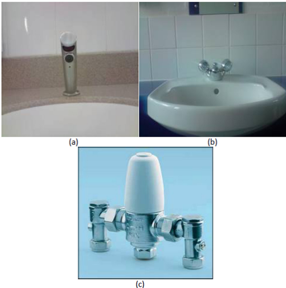
Fig. 1. (a) Electronic tap, (b) conventional mixer tap, and (c) thermostatic mixer valve.
