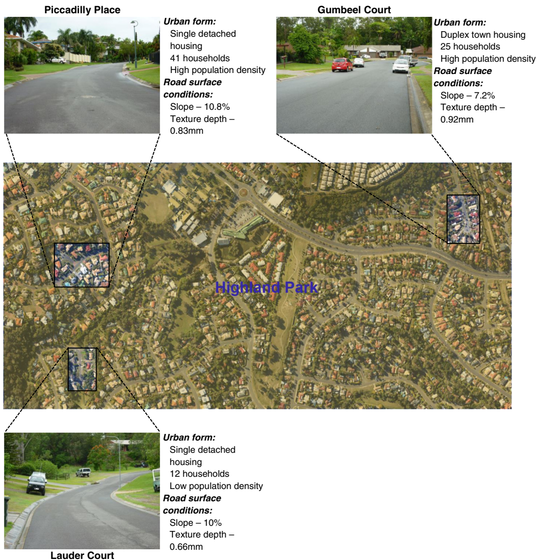
Fig. 1. Aerial and street views of study site locations in Highland Park Catchment.
