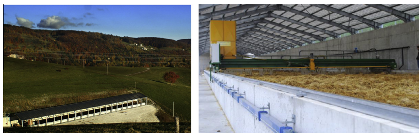
Fig. 1. Panoramic and detailed views of the treatment plant (photo: A. Chiumenti).
