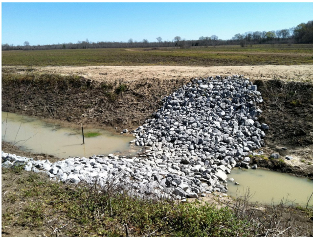
Fig. 1. Low-grade weir in a field setting.
