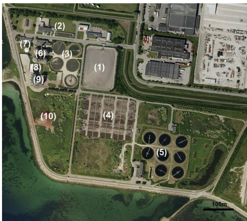
Fig. 1 – Aerial photo of the Avedøre WWTP (Map data: Google, Aerodata International Surveys). Numbers correspond to the description in the Section 2.1.
