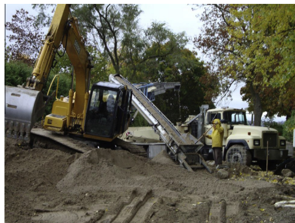
Fig. 2. A typical single-lot construction site in Southern Ontario.
