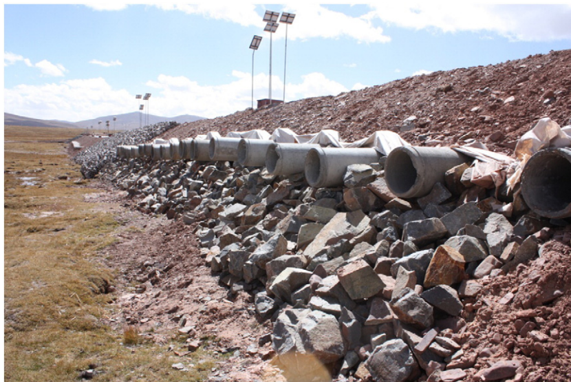
Fig. 1. A picture of the in-situ combined crushed-rock interlayer and ventilated ducts embankment.
