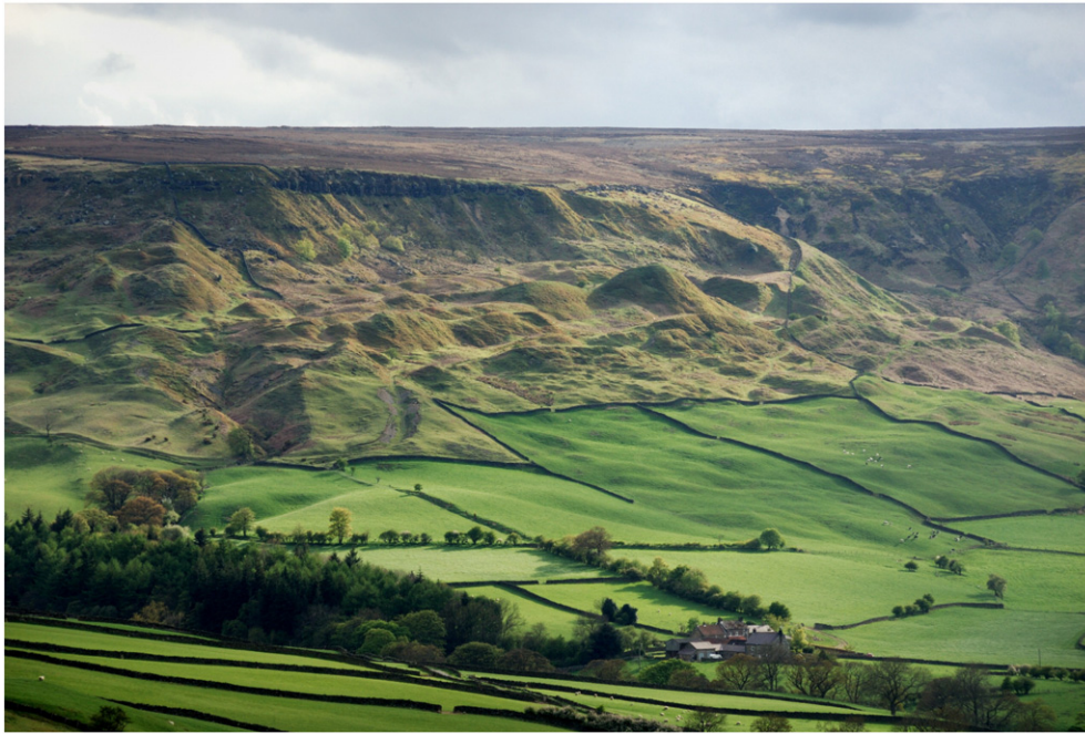
Fig. 1. The Mark Nab landslide on the Jurassic escarpment, showing complex landslide morphology. Looking south-west. Photo taken by A. H. Cooper. Copyright BGS/NERC P769517.
