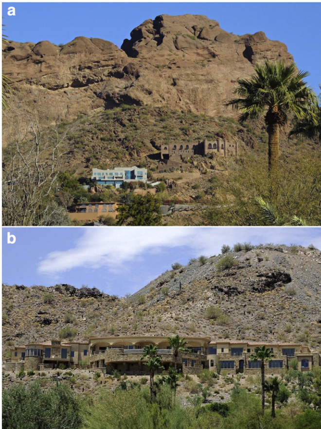
Fig. 1. Urban infrastructure at the foot of desert mountains. Expansive homes, water towers and other urban features often occur directly at the base of steep mountain slopes, exemplified here for mansions in (a) Phoenix and (b) Paradise Valley locations in central Arizona. Note construction of mansions on (a) a talus cone and (b) underneath scree.
