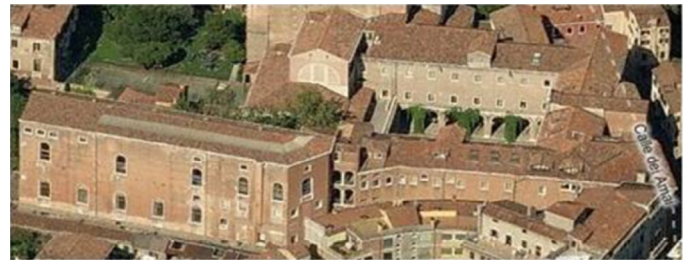
Fig. 1. Aerial photo of the Tolentini structure. (a) Longitudinal section. (b) Cross sections.
