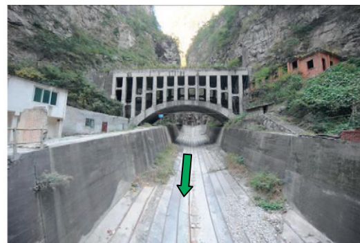
(b) V-type drainage channel
