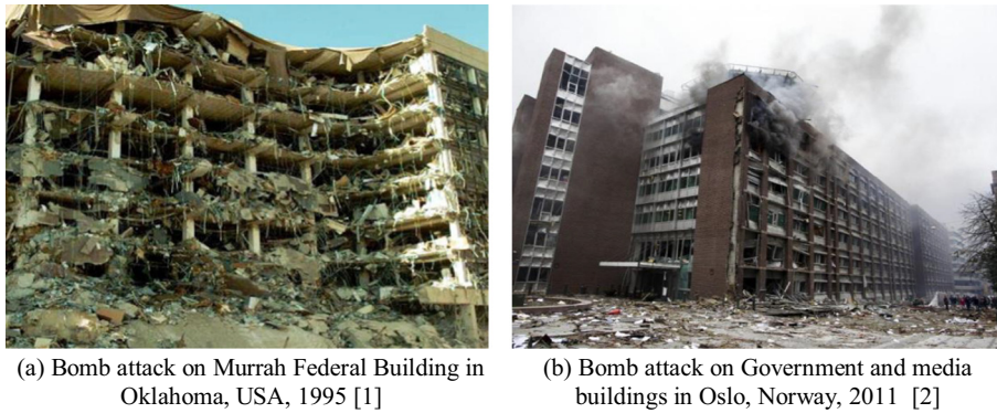
Fig. 1. Damage to the glazed facades from major bomb attacks.
