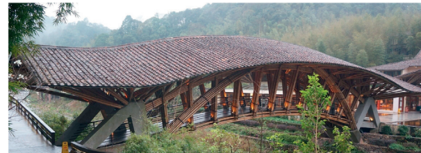
(a) Bamboo footbridge
