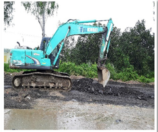
Fig. 1. Milling using Ripping & Crushing.
