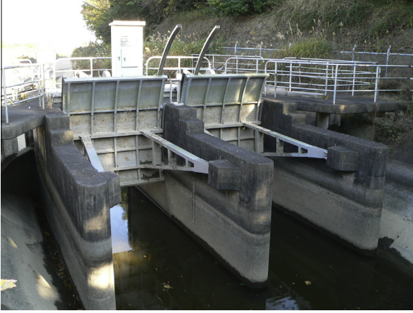
Fig. 1. Fully-opened radial gates along the Toyohashi-Tahara aqueduct, Toyohashi City (Japan) on 26 November 1998.
