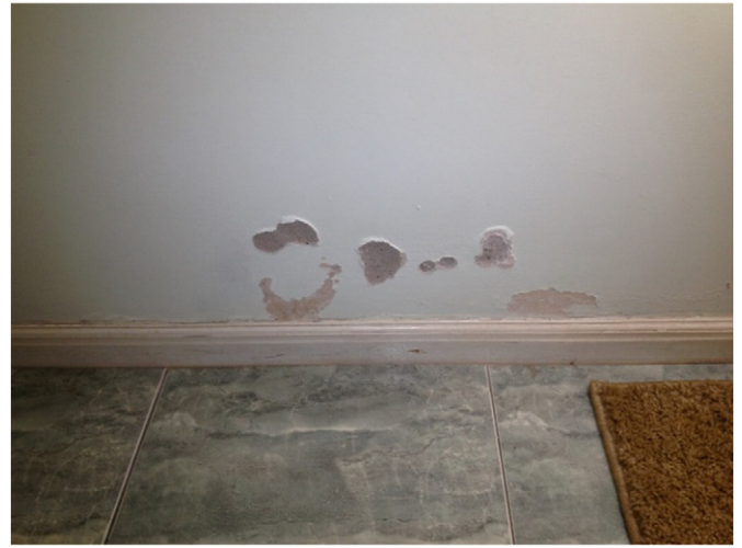
Fig. 2. Structural damage at a lower corner surface due to rising damp effect.
