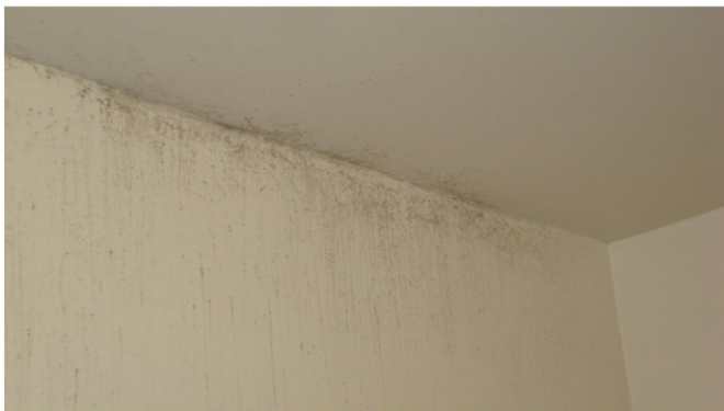
Fig. 1. Mold growth around an upper corner edge.
