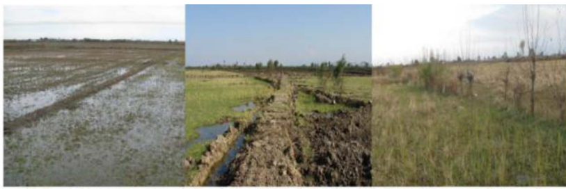
Lack of drainage, inappropriate road situation and boundary, before land development and renovation project
