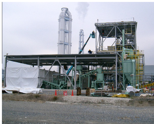
Fig. 1. Entrained-flow gasifier test plant (2 ton/day) at Kawagoe, Japan.
