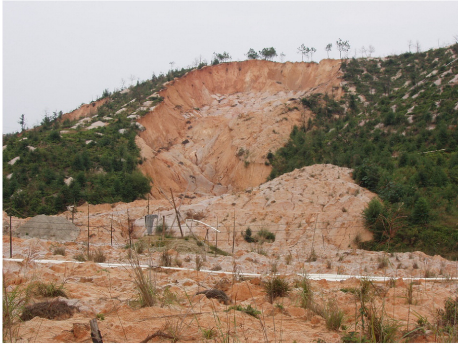
Fig. 1. The landslide caused by injection improperly.
