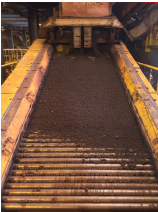
Fig. 1. Roller screen in operation.
