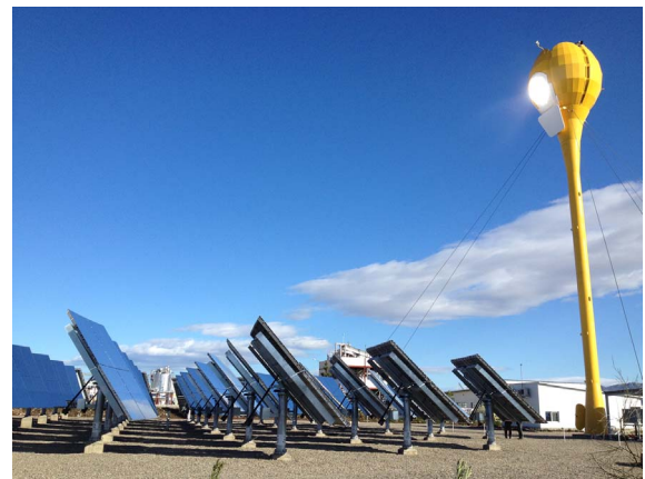
Fig. 1. Pilot plant CSP system with solarized CHP microturbine developed by AORA Solar Ltd [34].
