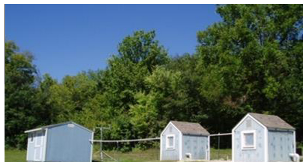
Fig. 1. Test houses (southeast view).
