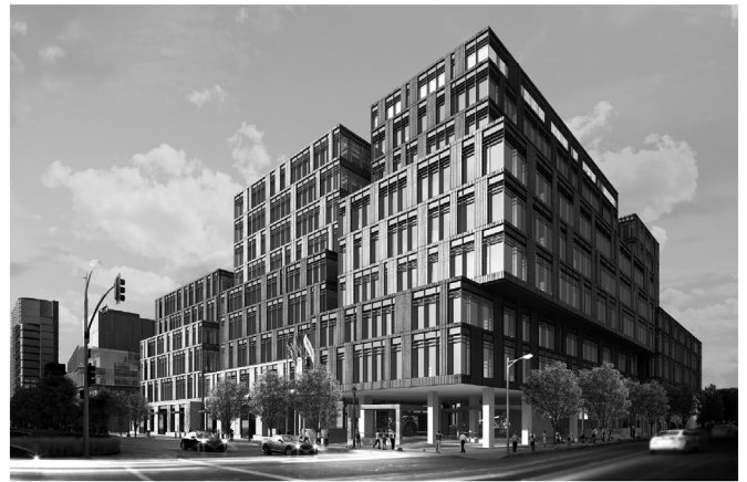
Fig. 1. Case study building.
