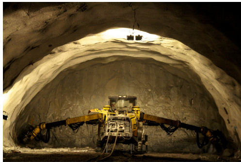
(a) Jumbo and excavation front
