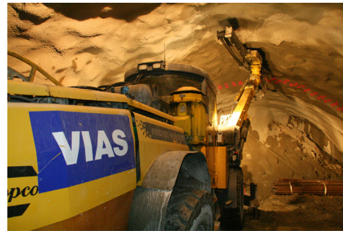
(b) Jumbo drilling holes on the excavation front
