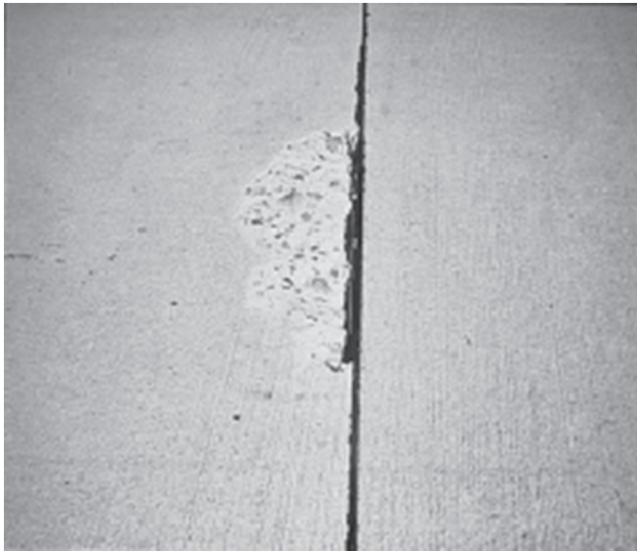
Fig. 1. Representative spall damage on the edge of a concrete slab [7].
