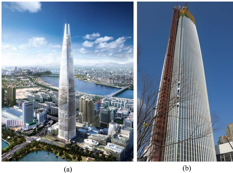
Fig. 1. The LWT: (a) Perspective view of the LWT, (b) the LWT under construction (February 2015).
