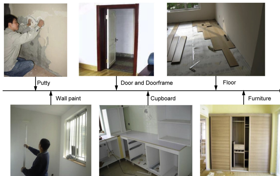
Fig. 1. A typical interior construction process in China related to VOC emissions.
