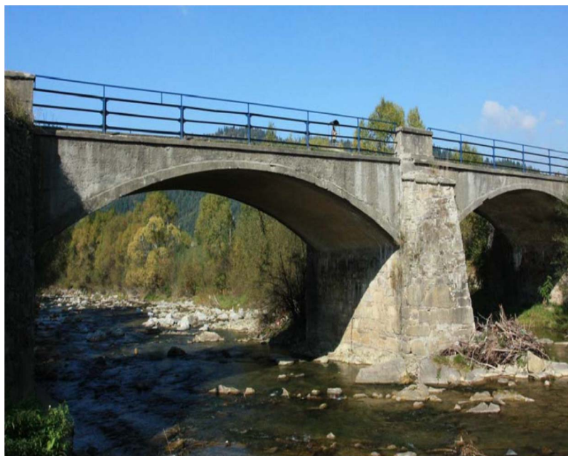
Fig. 1. Reinforced concrete bridge Krásno nad Kysucou before reconstruction in 2014.
