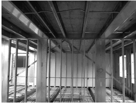
Fig. 1. Concrete-filled light gauge steel composite columns imbedded within prefabricated modular walls [1].
