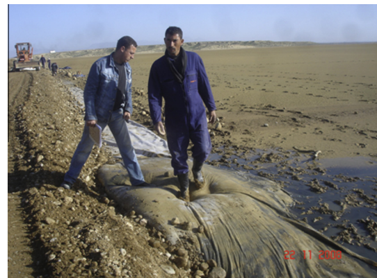
Fig. 3. Embankment over locally weak zone.
