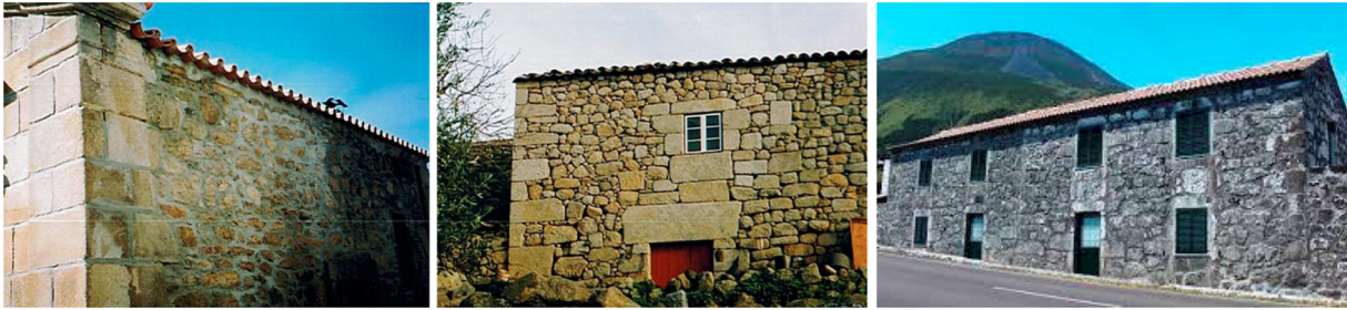
Fig. 1. Example of typical Portuguese stone masonry constructions.
